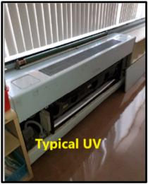
The existing unit ventilators are original to the age of the building. The main components of the unit ventilator are fan, hot water coil, and air damper to control outside and return air. During the
