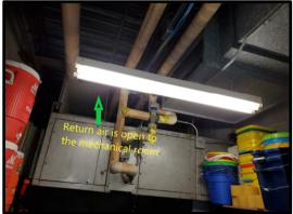
Two air-handling units serve the gymnasium area. Both units are operated by pneumatic controls. During the walkthrough, we noticed that return air for the AHU is open to the mechanical room, and it is not connected to the return air duct. This arrangement
