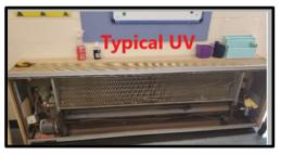
The existing unit ventilators are original to the age of the building. There are 13 unit ventilators in the building. The main components of a unit ventilator are a fan, steam coil, and air damper to control outside and return air. During the walk-through, we noticed that air damper was closed for outside air, so the unit was recirculating 100% room air in the space. According to facility personnel, the outside air is controlled by
