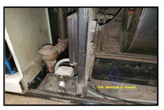
walk-through, we noticed that the air damper was closed for outside air, so the unit was recirculating 100% room air in the space. According to facility personnel, the outside air is controlled by a
