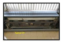
The existing unit ventilators are original to the building. Similar to the other schools, the outside air damper was closed for outside air, so the unit was recirculating 100% room air in the space. Current Classroom unit ventilators are capable of providing ventilation (with manual changes) with proper adjustment of pneumatic control inside
